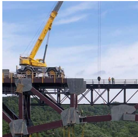
A bridge under construction in New York. Photo courtesy of Norfolk Southern.
