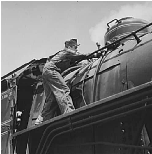
Tennessee Valley Authority. Railroad crews at Watts Bar Dam. Clearing the sand line is one of the chores that fall to the “tallow pot,” or fireman, of a railway locomotive. In addition to jobs like this, the “tallow pot” serves up an average of eight to ten tons of coal each eight hour day to the big “hog,” or locomotive.
