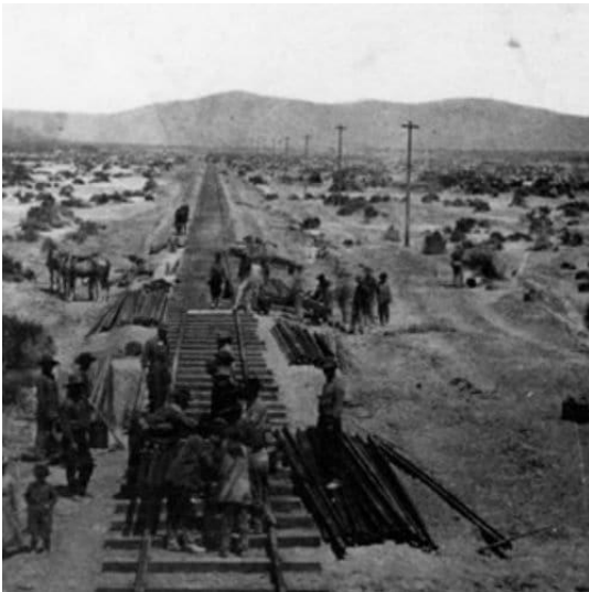
Central Pacific workers lay rail at the end of track, Humboldt Plains, Nevada. 1868. Courtesy of The Bancroft Library, University of California, Berkeley.
