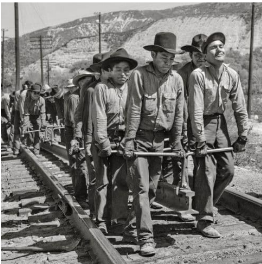
Rail workers manually move one piece of rail. March 1943. Photo by Jack Delano, Office of War Information.
