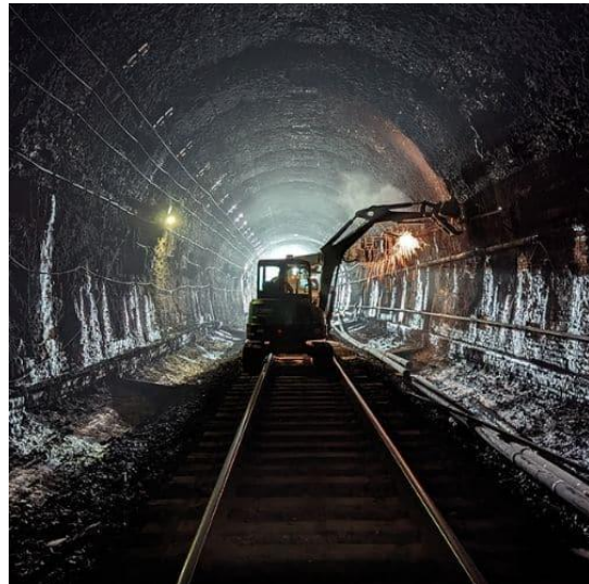
One example of the many investments Class I railroads make: CSX reopened the expanded Howard Street Tunnel in fall 2025, removing a major East Coast bottleneck and paving the way for double-stack container trains through Baltimore.
