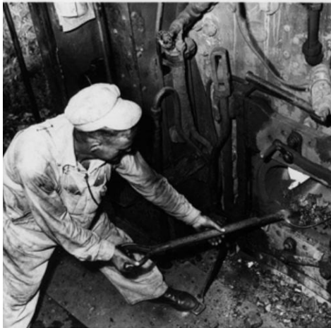
Before: Firemen did the difficult work of continually stoking the locomotive firebox. ( Photo Source )
