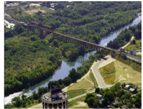
Laredo International Rail Bridge with Mexico on the left and the U.S. on the right. Photo credit: FRA.
